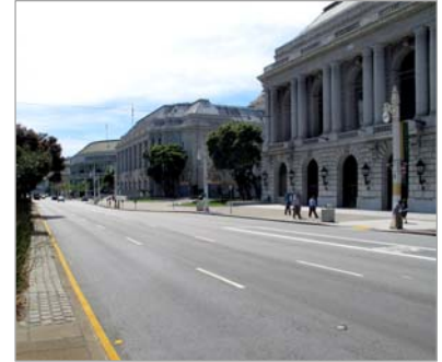
The rear façade of City Hall faces Van Ness Avenue, across from the San Francisco War Memorial and Performing Arts Center.
