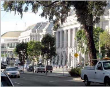
While most blocks of Van Ness Avenue feature a consistent row of sidewalk trees of varied type and maturity, the presence of trees in the median is less consistent throughout the corridor.
