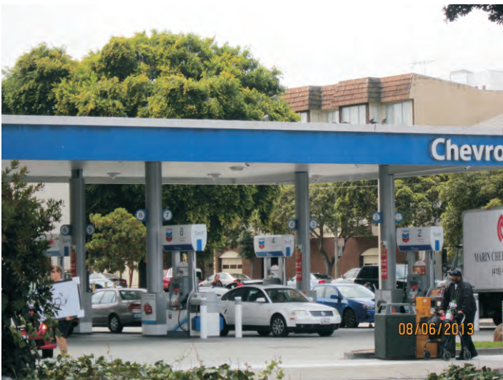
Site 27: Chevron, 3675 Geary Boulevard.
