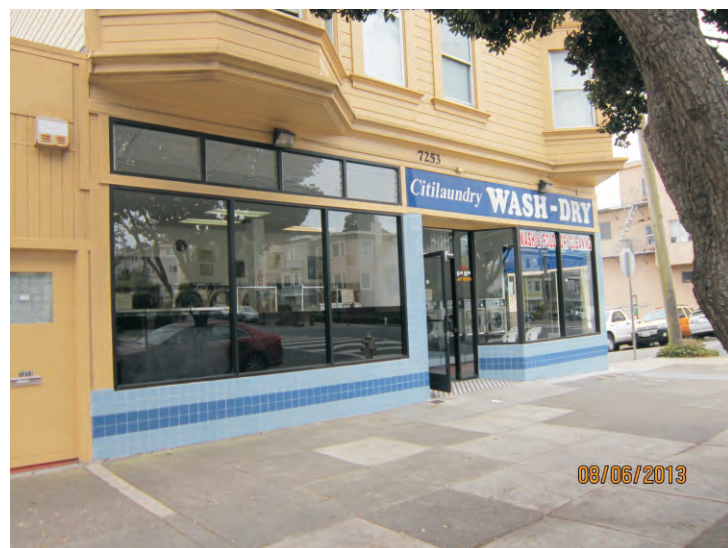
Site 44: Citilaundry, 7253 Geary Boulevard.
