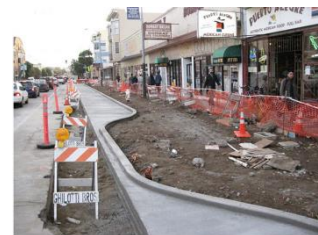
Sidewalk conditions during pavement and sidewalk repair
