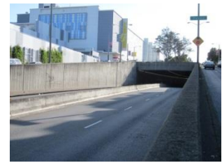
Westbound view of the existing Masonic tunnel.
