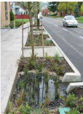
Tree Basin - an example of LID that allows stormwater runoff to infiltrate into the soil, thereby reducing runoff volume and peak flows.
