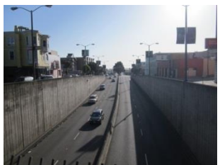
Looking west from atop the Masonic tunnel.
