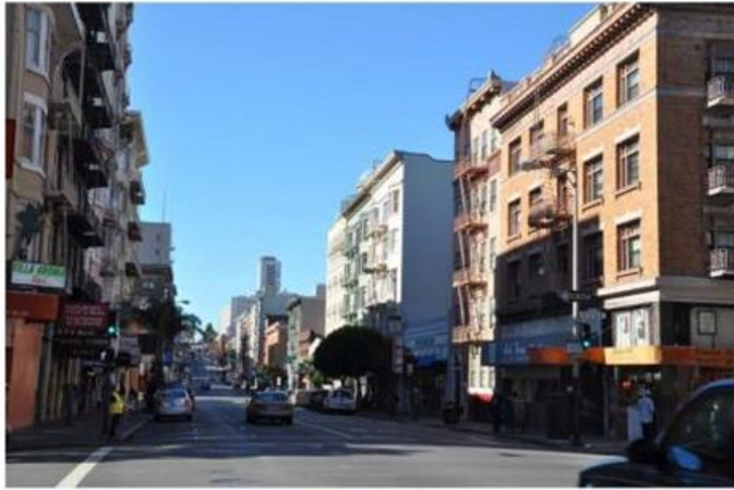
a. Typical Tenderloin 2 – 5-story masonry residential streetscape.
