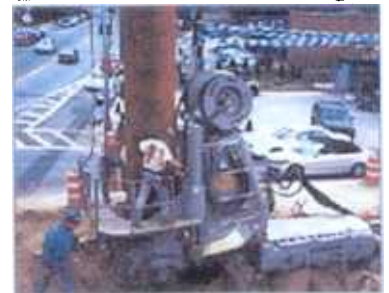
Piling Work beside Traffic
