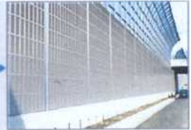
Noise barrier panels attached to the GIKEN WALL
