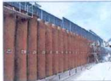
The GIKEN WALL as seen after excavation work.
