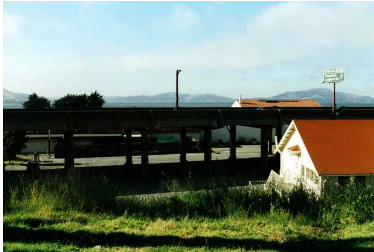
Viewpoint 5 – From the Former Burger King (Building 211)
