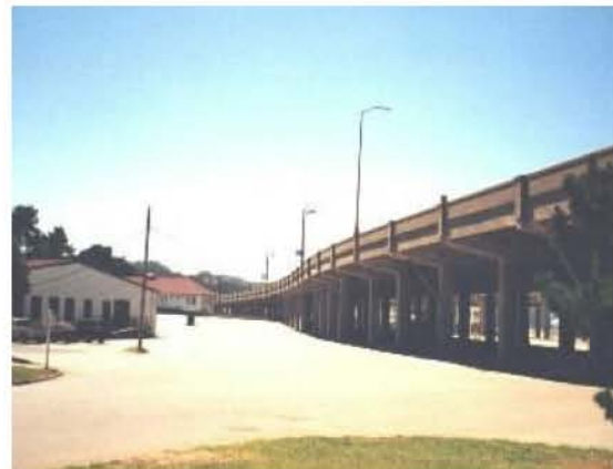
Main Post Landscape Unit
