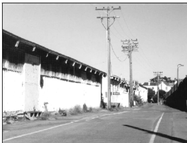
Buildings 1184, 1183, and 1182, camera facing east.
