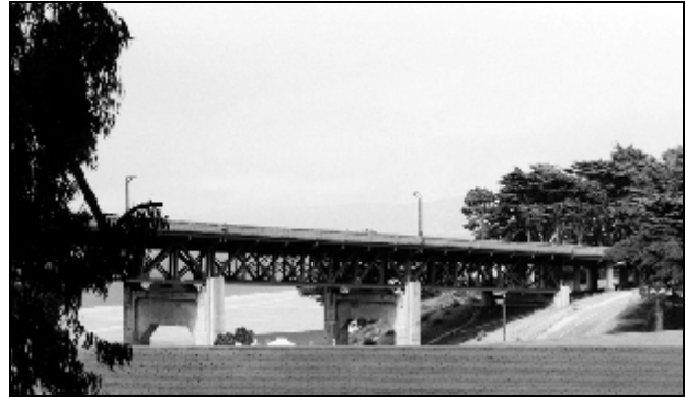
Doyle Drive viaduct structure
