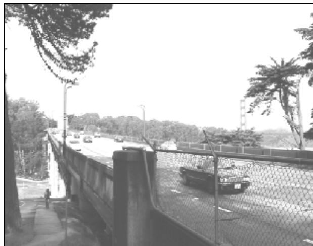
Doyle Drive with the Golden Gate Bridge in the background.
