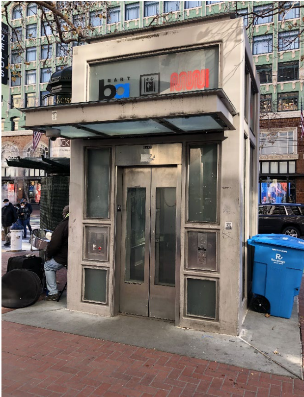
Figure 5. Street elevator at Powell St. Station, December 2021.
