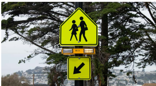
Crosswalk warning signs with flashing lights to increase pedestrian visibility by alerting drivers to yield to people crossing the street.
