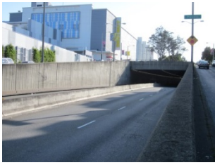
Westbound view of the existing Masonic tunnel.
