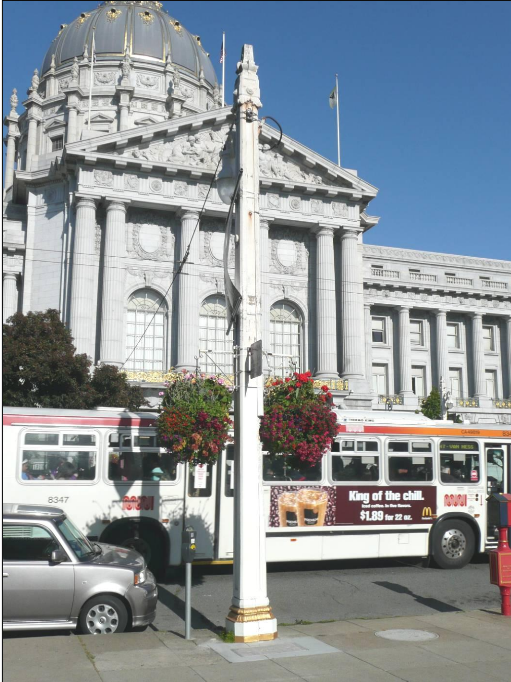
Photograph 11: Exterior wiring, signage, and flower baskets on Pole 41, showing gold paint on original base, between McAllister Street and Grove Street, 4/1/2009.
