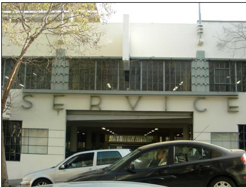
Photograph 4: 945-999 Van Ness Avenue, service entry, camera facing south, 3/8/09
