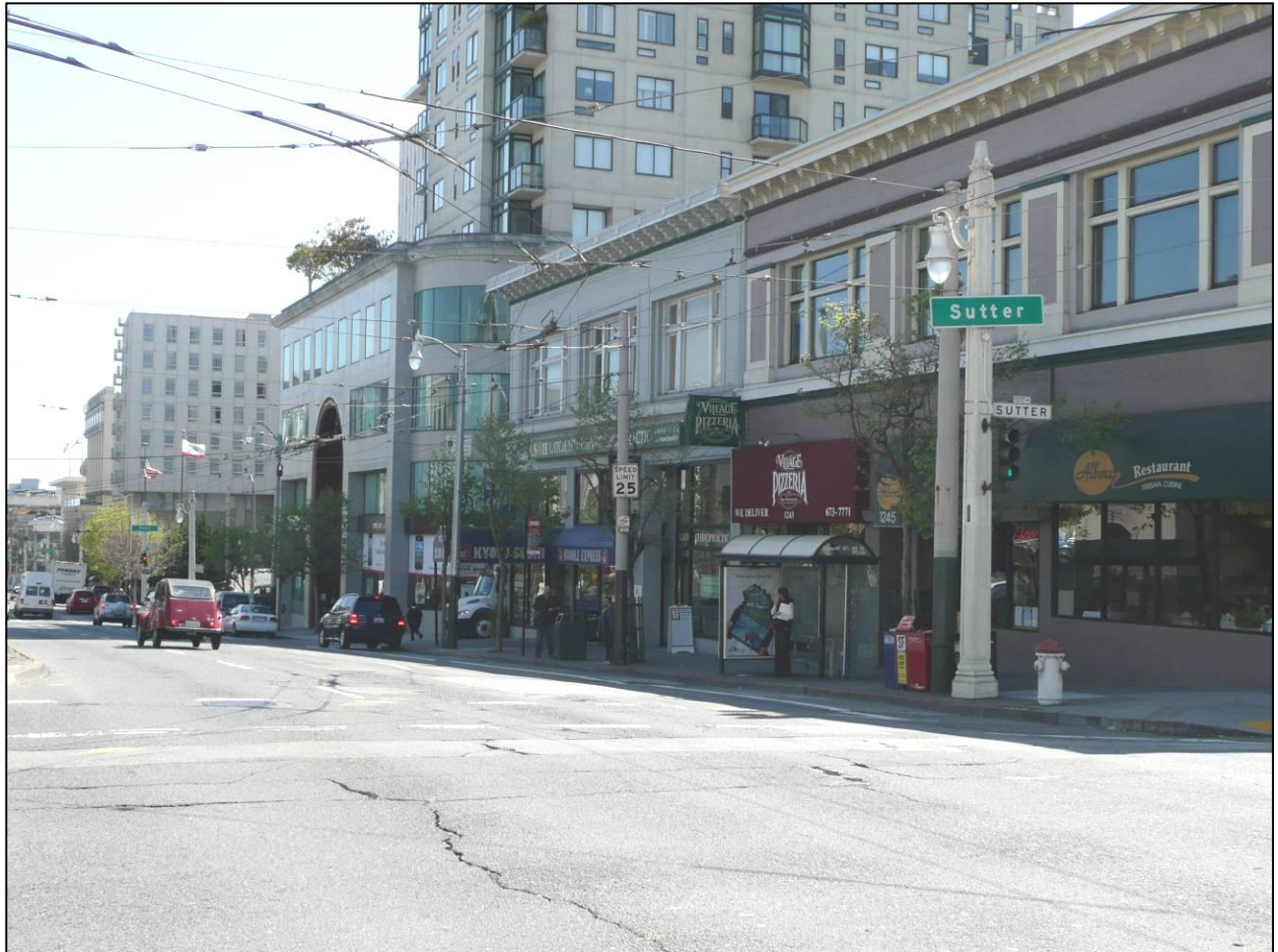
Photograph 14: Block between Sutter Street and Post Street, showing missing poles replaced by modern metal poles, 4/1/2009.
