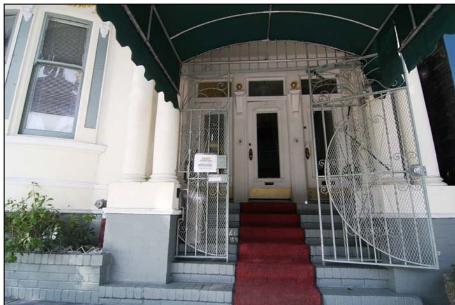
Photograph 3: 2517-2521 Van Ness Avenue, entry detail, camera facing west, 3/8/09
