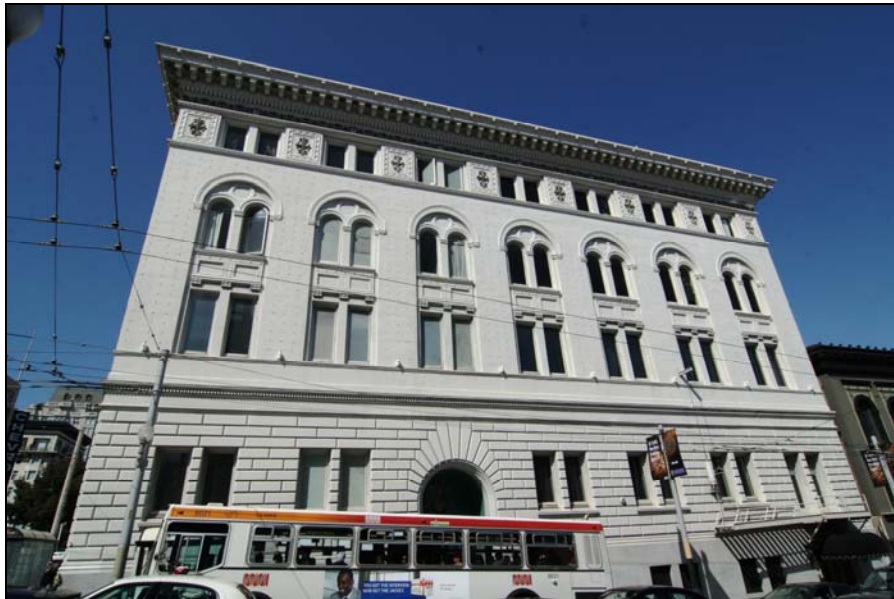
Photograph 3 : 1320 Van Ness Avenue, camera facing east, 3/8/09
