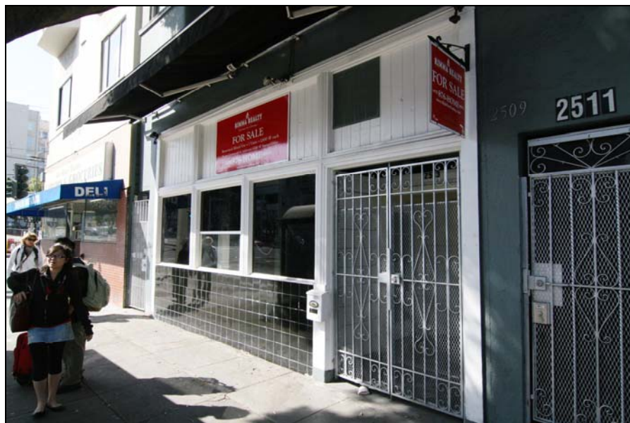
Photograph 2: 2509-2515 Van Ness Avenue, storefront detail, camera facing southwest, 3/8/09
