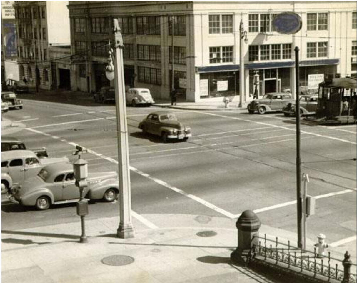
Photograph 20: Trolley Poles with 1936 light fixtures at Van Ness Avenue and O'Farrell Street, as of 1943, (Pole 101 in foreground and Pole 98 in background at diagonal, camera facing southeast). See current pole condition in Photograph 21 below. Photograph courtesy of San Francisco Public Library Historical Photograph Collection.
