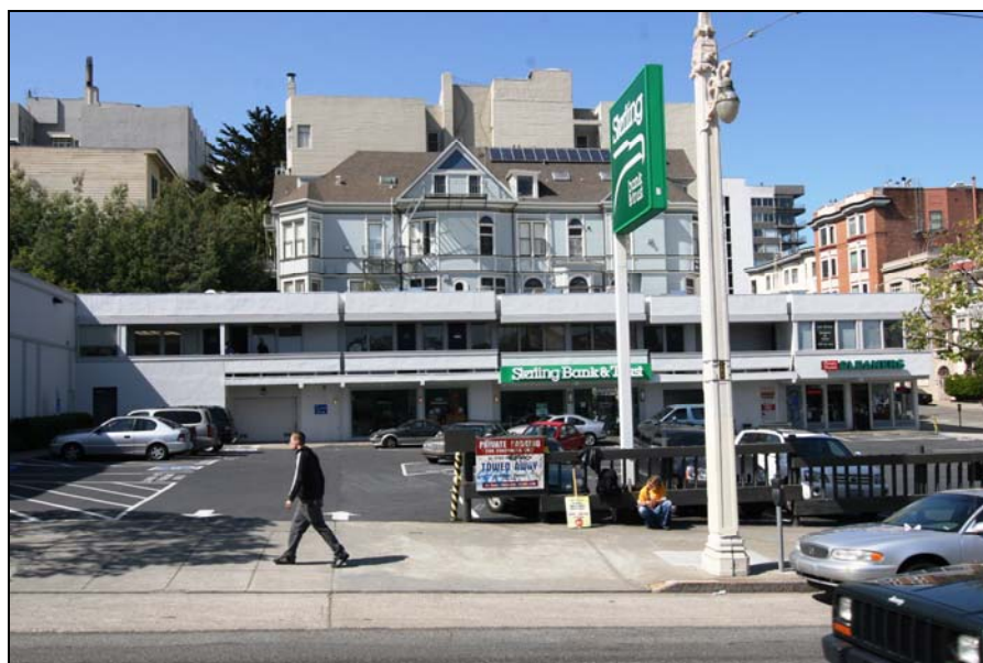
Photograph 3: 207 Van Ness Avenue, addition, camera facing west, 3/8/09
