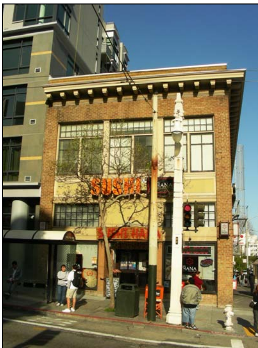
Photograph 2: 800 Van Ness Avenue, camera facing east, 3/8/09
