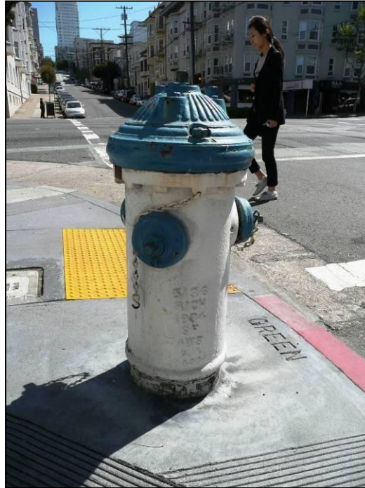
Photograph 9: Hydrant at Van Ness Avenue and Green Street, 3/9/09.
