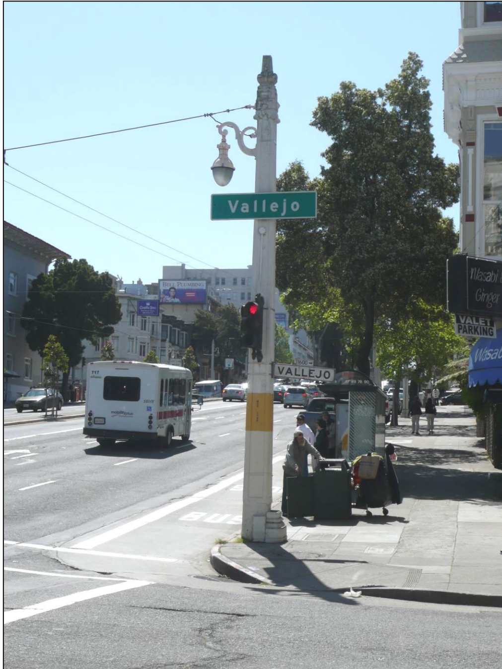
Photograph 6: Partial base, traffic signal equipment inserted, and signage on Pole 227, southwest corner of Van Ness Avenue and Vallejo Street, 4/1/2009.
