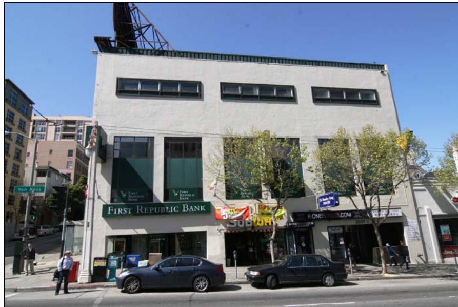
Photograph 2: 2001 Van Ness Avenue, camera facing west, 3/8/09
