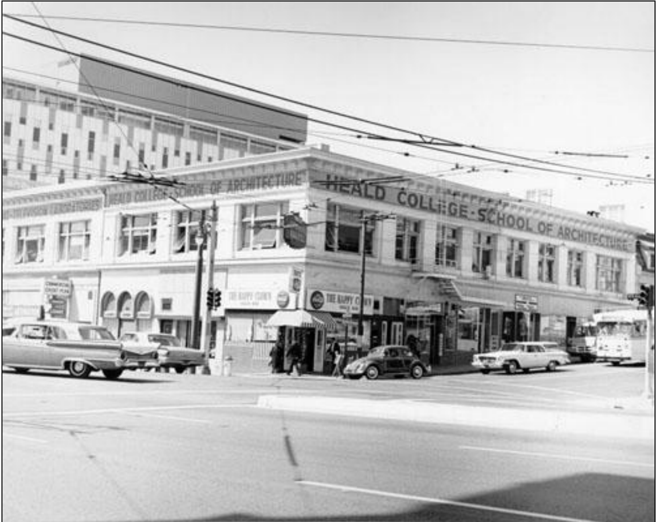
Photograph 23: Pole 127, Van Ness Avenue and Sutter Street, as of 1964. Traffic signal equipment has been inserted in the pole and a modern metal pole installed immediately adjacent. Photograph courtesy of San Francisco Public Library Historical Photograph Collection.
