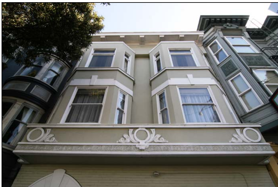
Photograph 3: 2430 Van Ness Avenue, detail of stacked bays, camera facing east, 3/8/09
