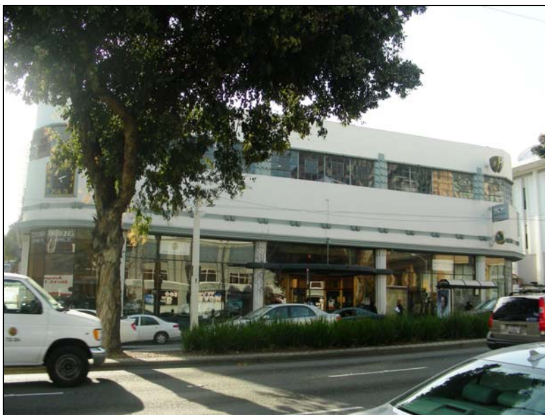
Photograph 5: 945-999 Van Ness Avenue, central customer entry, camera facing west, 3/8/09
