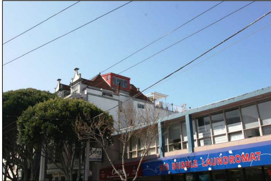
Photograph 2: 2517-2521 Van Ness Avenue, rooftop addition, camera facing southwest, 3/8/09
