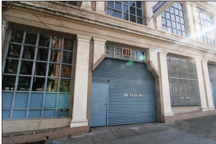
Photograph 4: 799 Van Ness Avenue, secondary garage entry, camera facing south, 3/8/09
