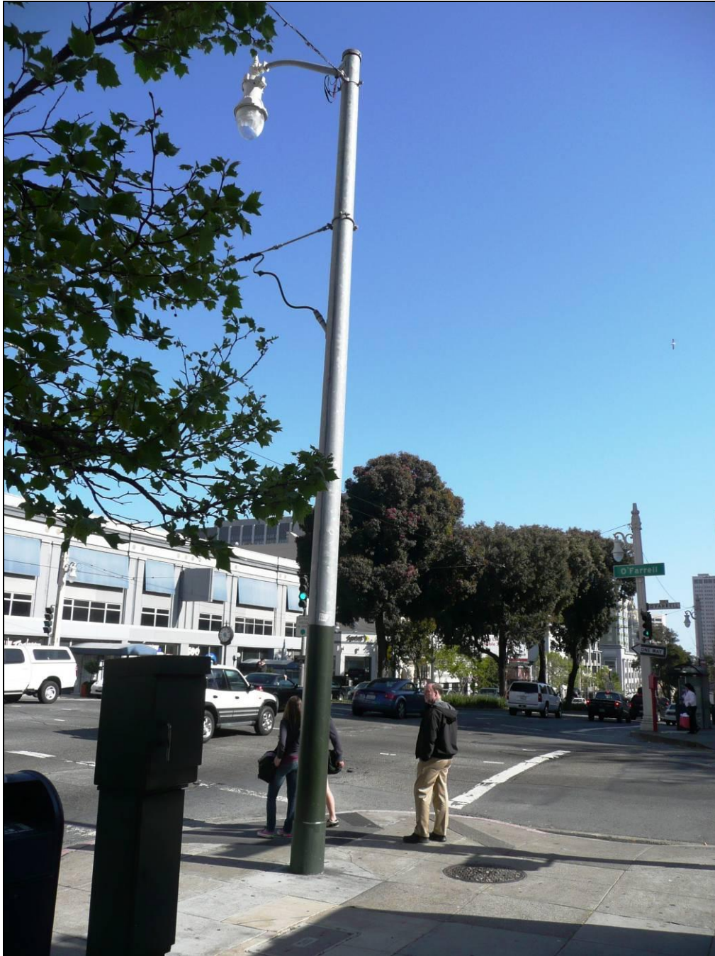
Photograph 21: Replacement metal pole in location of Pole 101, Van Ness Avenue and O'Farrell Street, 4/1/2009 (shown in Photograph 20 above).
