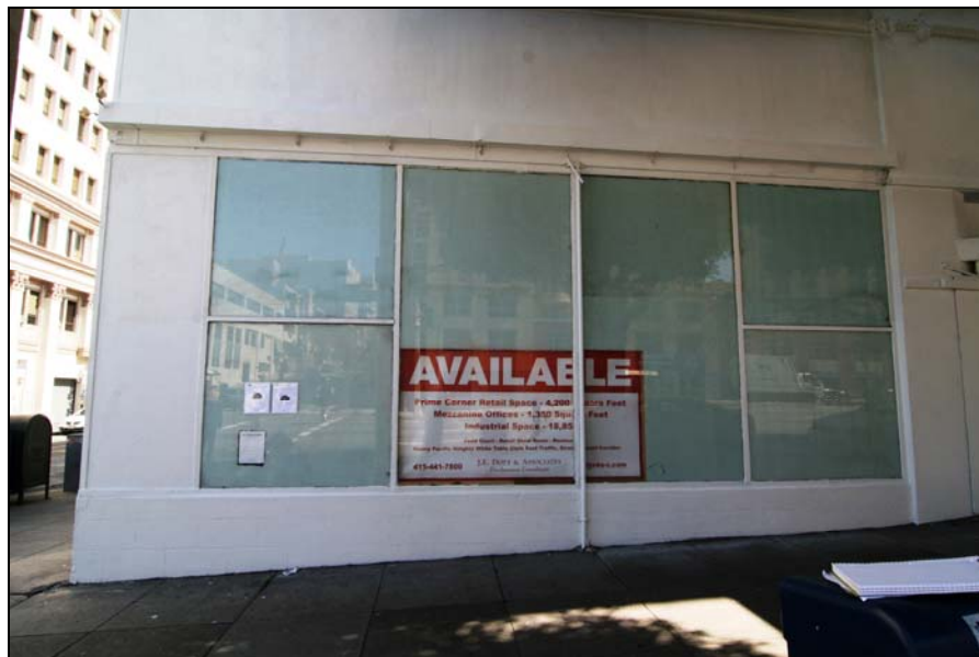
Photograph 5: 1946 Van Ness Avenue, steel frame display window on Van Ness Avenue, 3/8/09
