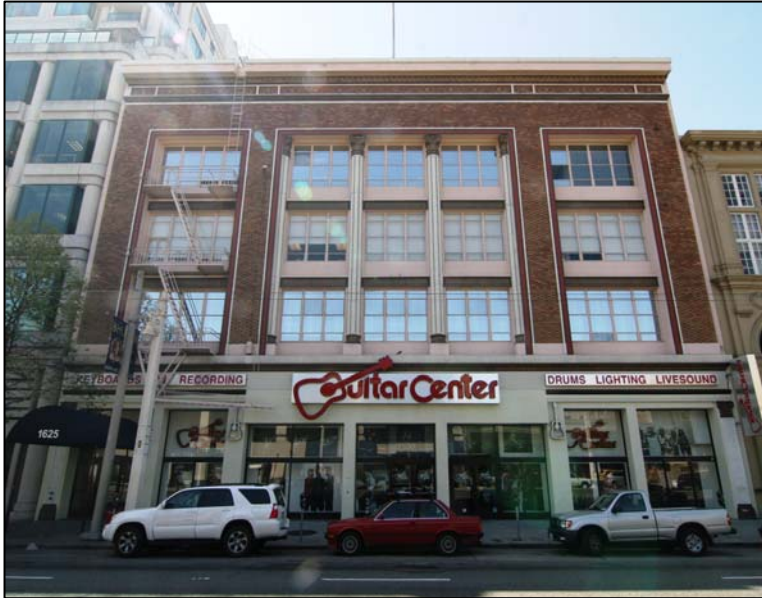
Photograph 1: 1625 Van Ness Avenue Van Ness façade, camera facing west, 3/8/09
