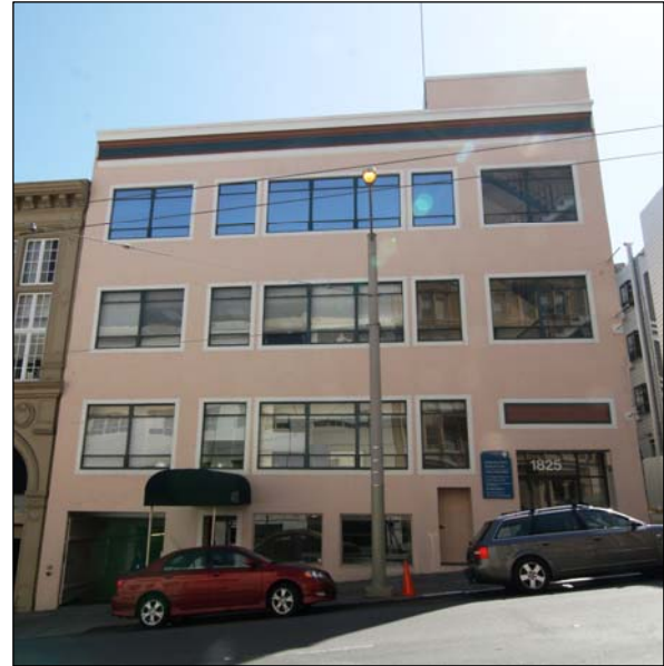
Photograph 2: 1625 Van Ness Avenue Sacramento Street façade, camera facing south, 3/8/09
