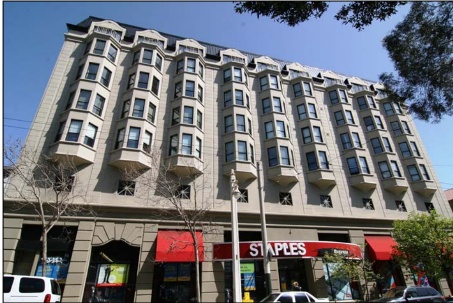
Photograph 2: 1776 Sacramento Street, camera facing east, 3/8/09
