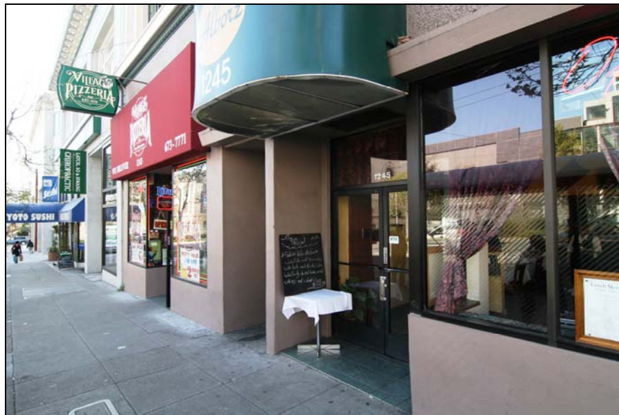
Photograph 3: 1243 Van Ness representative storefront insertion, camera facing southeast, 3/8/09
