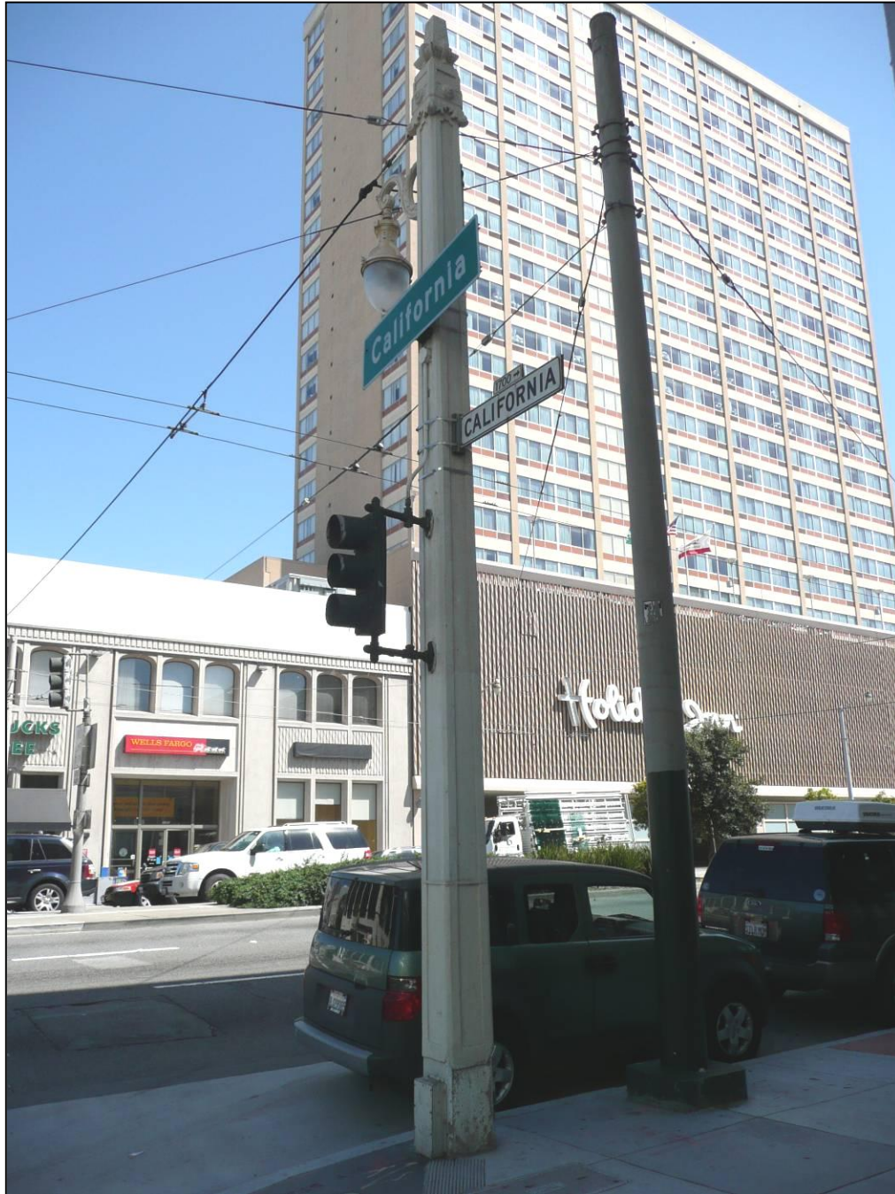
Photograph 12: Alterations to Pole 157, including insertion of traffic signal equipment, signage added, base removed, and modern metal pole installed adjacent. Located southwest corner of Van Ness Avenue and California Street, 4/1/2009.
