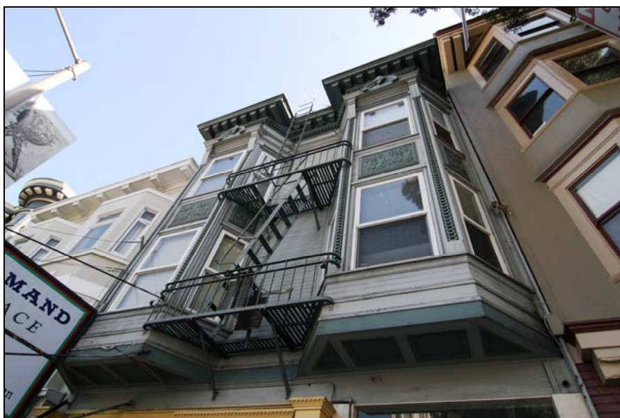
Photograph 3: 2420-2424 Van Ness Avenue, stacked bay detail, camera facing east, 3/8/09
