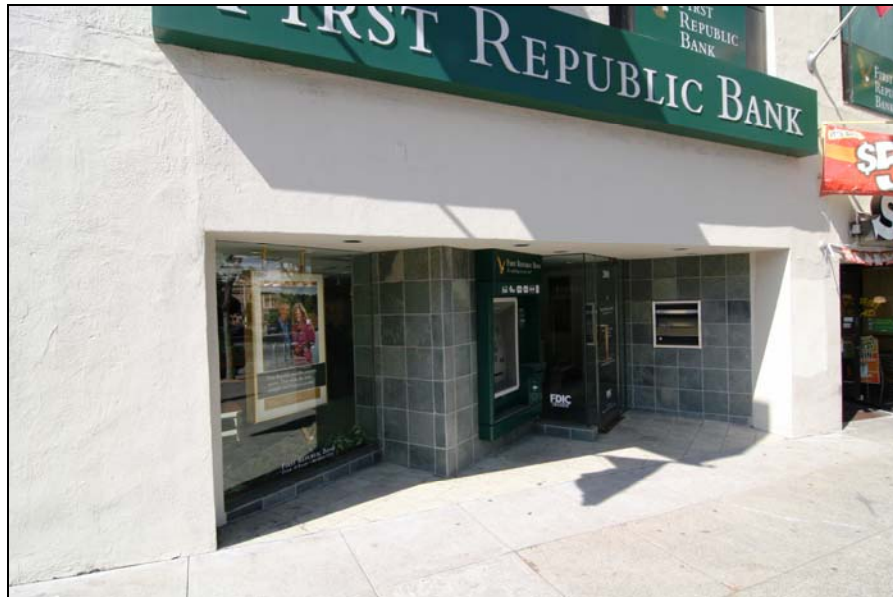
Photograph 3: 2001 Van Ness Avenue, storefront detail, camera facing northwest, 3/8/09
