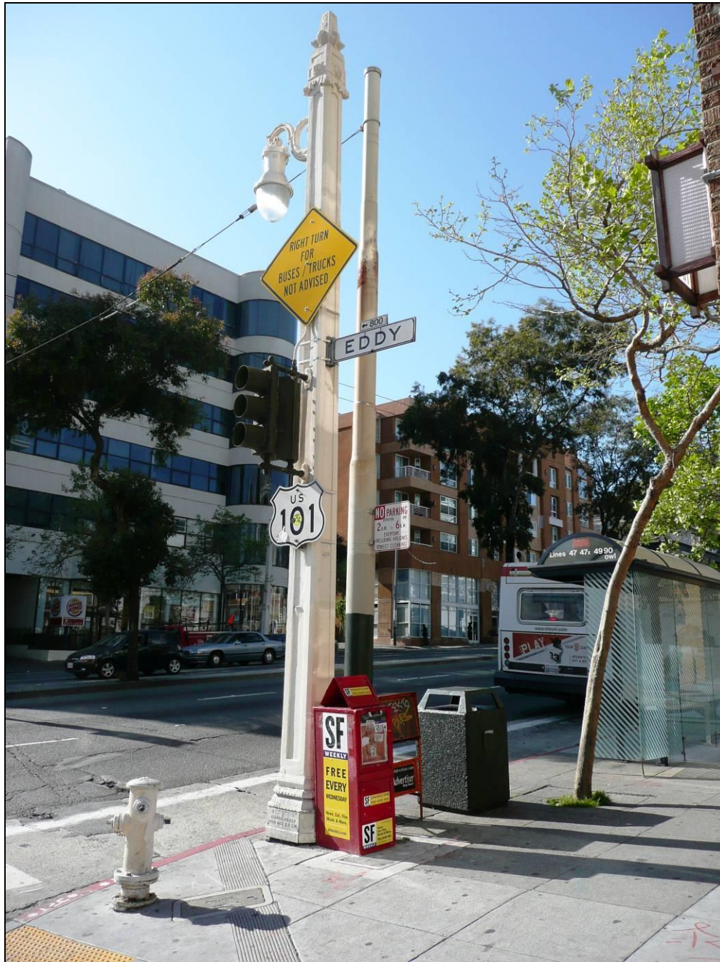
Photograph 17: Pole 82 with insertion of traffic signal equipment, signage added, and modern metal pole installed adjacent, Van Ness Avenue and Eddy Street, 4/1/2009 (shown in Photograph 16 above).
