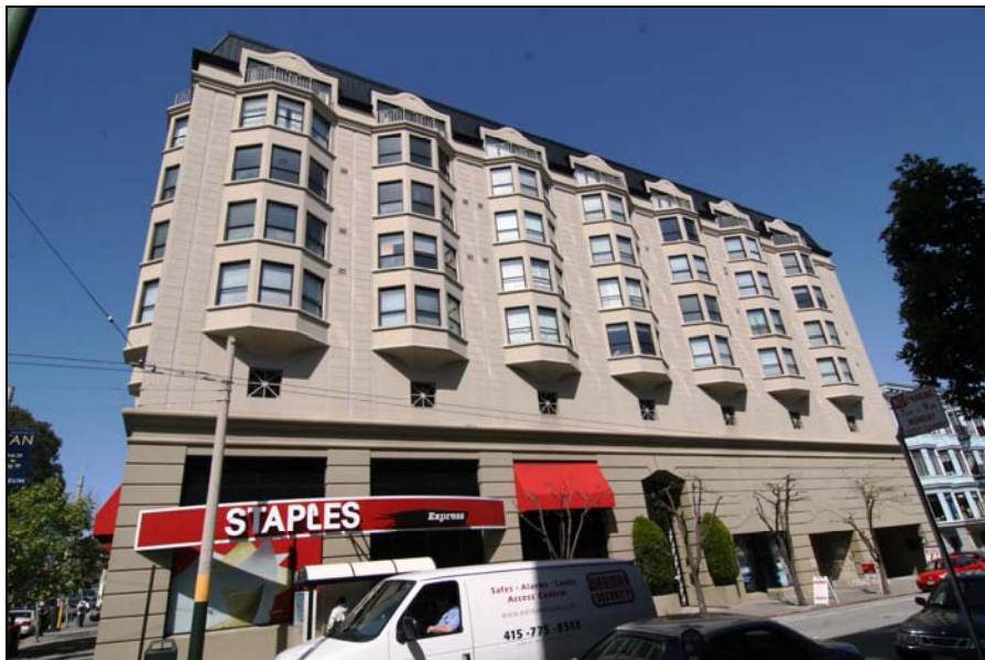
Photograph 3: 1776 Sacramento Street, camera facing north, 3/8/09
