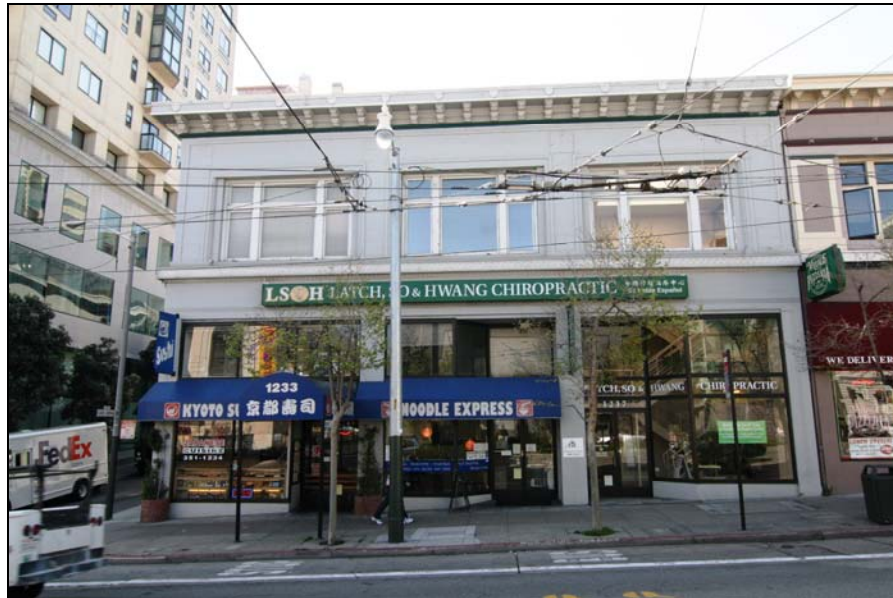
Photograph 2: 1233 Van Ness Avenue, camera facing west, 3/8/09
