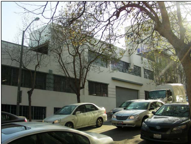
Photograph 3: 945-999 Van Ness Avenue, secondary elevation, camera facing southwest, 3/8/09
