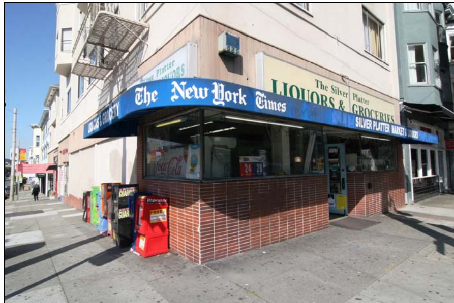
Photograph 2: 2501 Van Ness Avenue, storefront detail, camera facing northwest, 3/8/09
