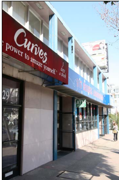
Photograph 2: 2525-2545 Van Ness Avenue, storefront detail, camera facing northwest, 3/8/09
