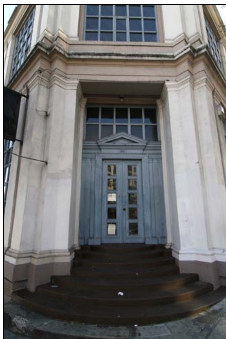
Photograph 3: 799 Van Ness Avenue, doorway detail, camera facing southwest, 3/8/09
