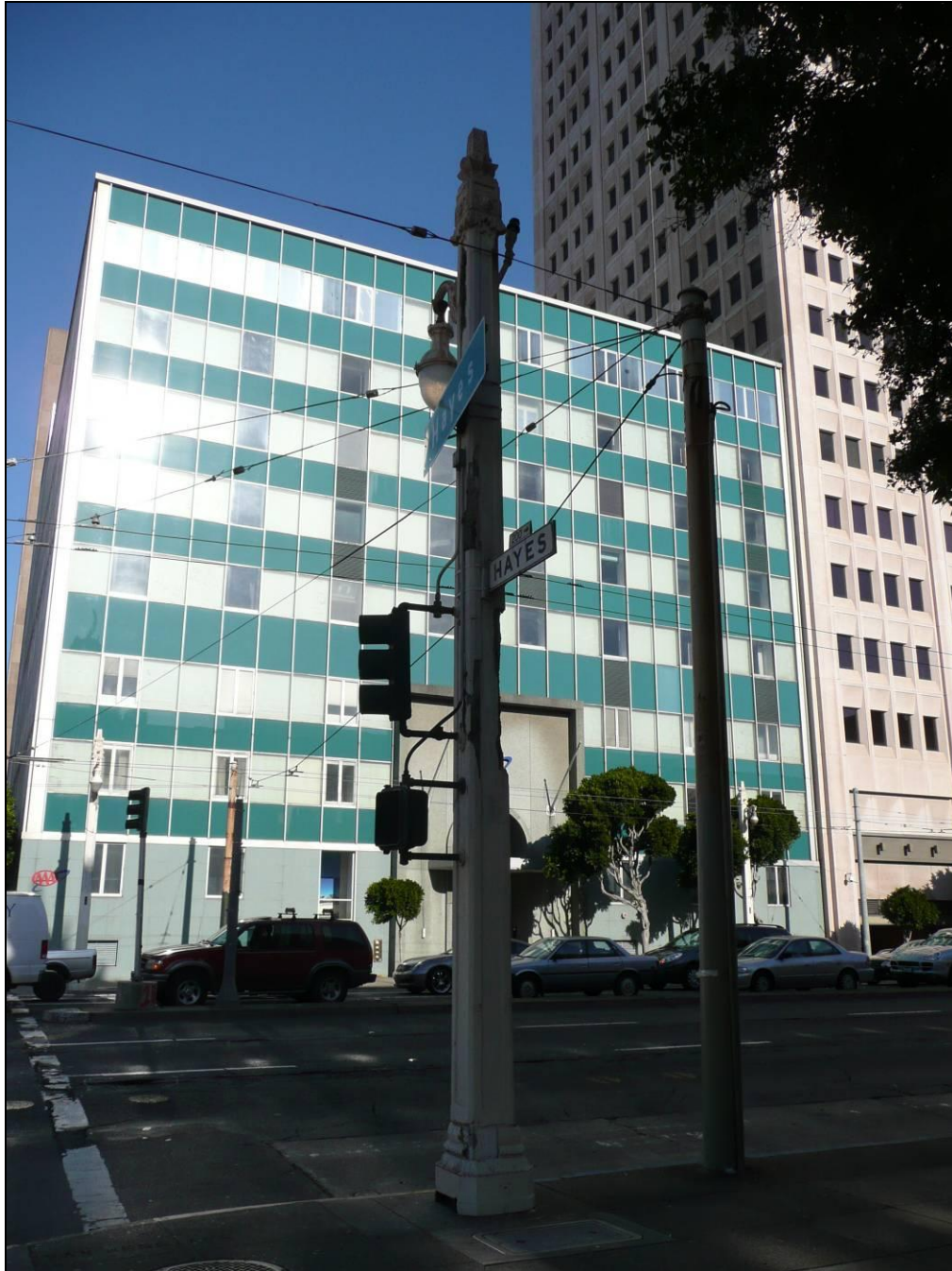
Photograph 19: Pole 17, with insertion of traffic signal equipment, signage added, and installation of adjacent modern metal pole, Van Ness Avenue and Hayes Street, 4/1/2009 (shown in Photograph 18 above).
