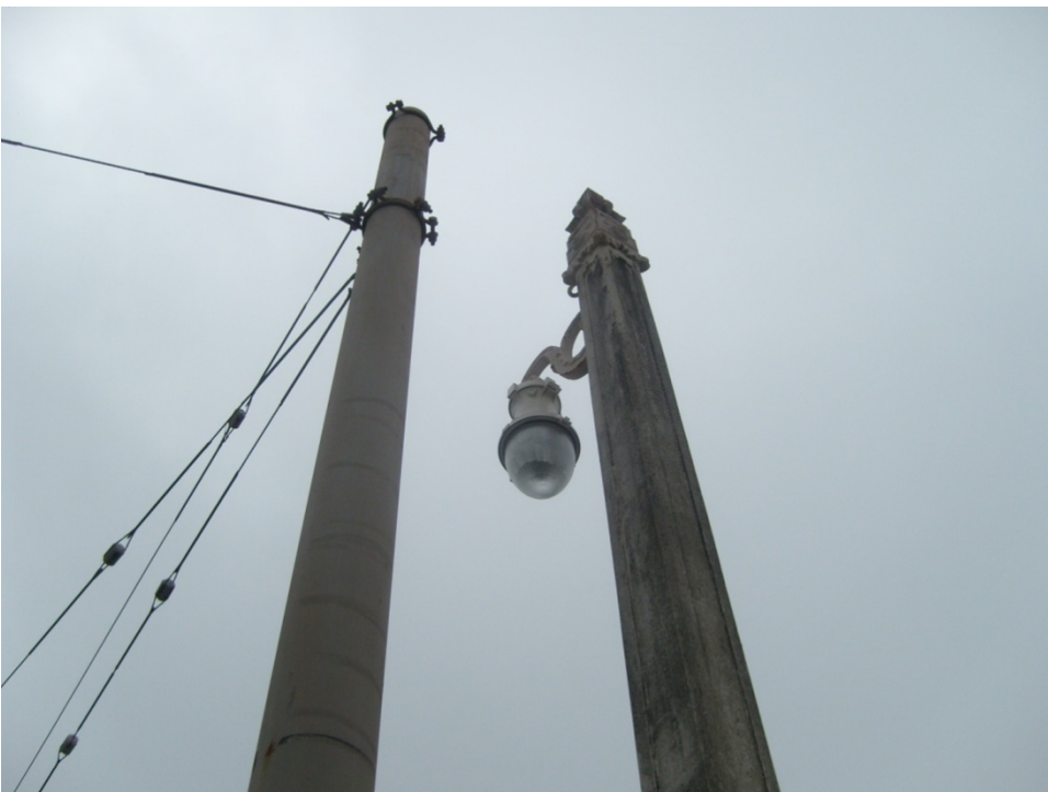
Figure 2.2: Supplementary Steel Pole, North Point and Van Ness Avenue (Pole 315)
