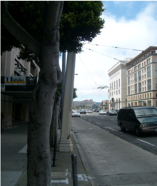
Figure 2.1: Out of Plumb, Fell and Van Ness Avenue (Pole 16)
