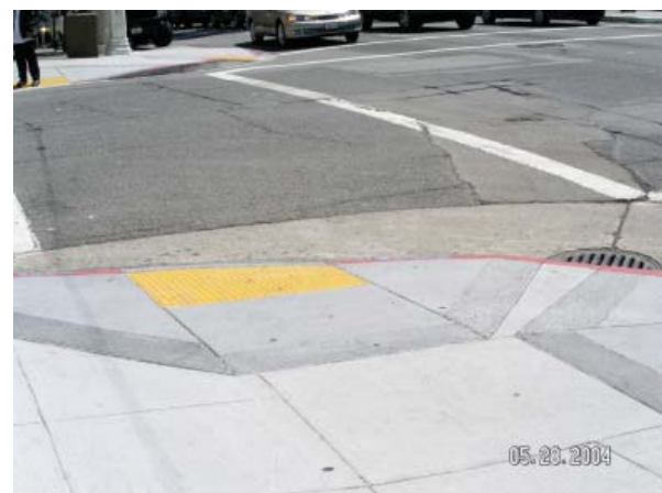
Figure 2-21: Recent Pedestrian Enhancements Installed on Van Ness Avenue
