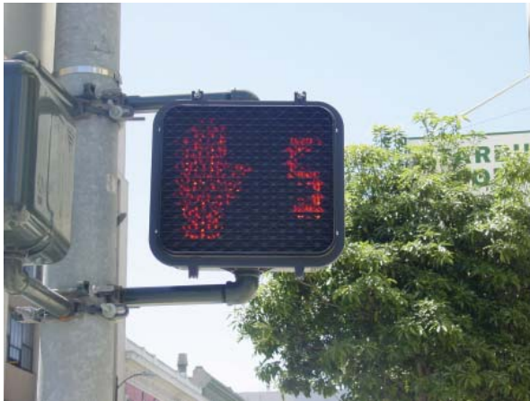
Figure 2-23: Countdown signals are found at some intersections
