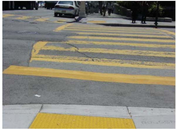
Figure 2-22: A visibly striped zebra crosswalk
