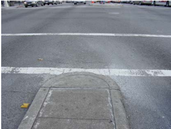
Figure 2-21: The tapered median at many intersections is not ideal as a pedestrian safety refuge
