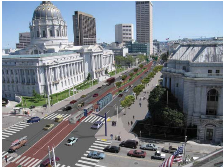
Figure 3-14: Alternative 4, Center Lane BRT with Side Platforms and Center Median, at City Hall
