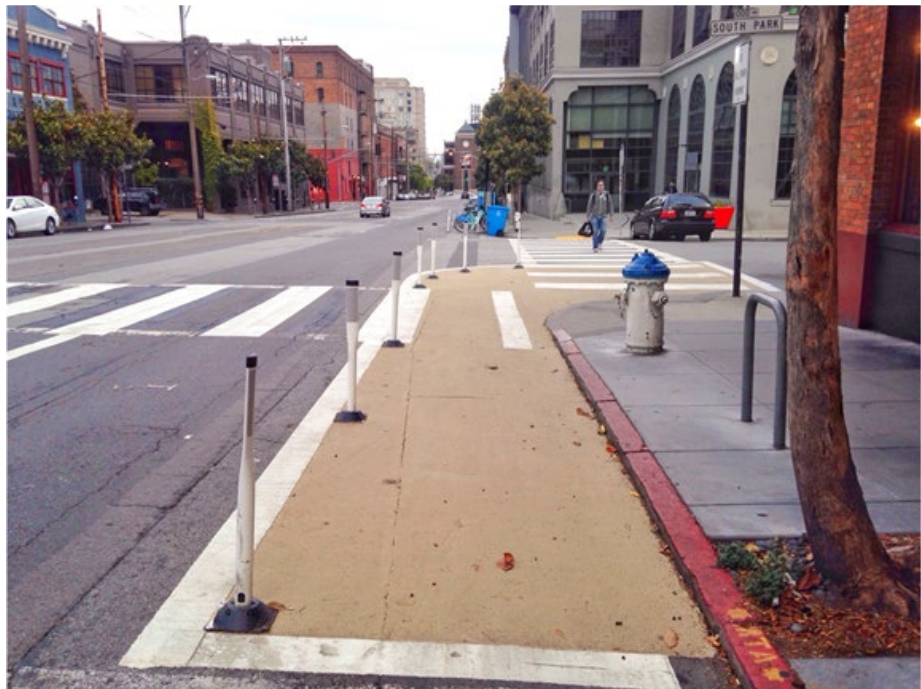
Typical Before – Painted Safety Zone
