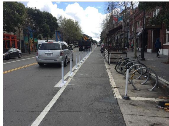
Figure 5: Valencia at 18th Street with new one-foot buffer and flex-posts
