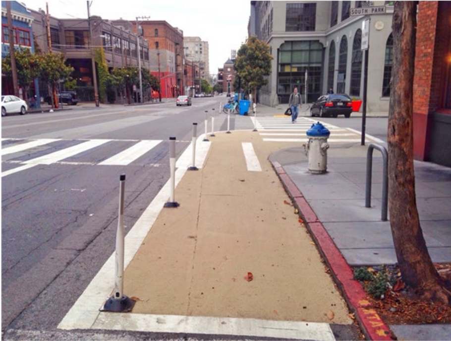
Typical Before – Painted Safety Zone
