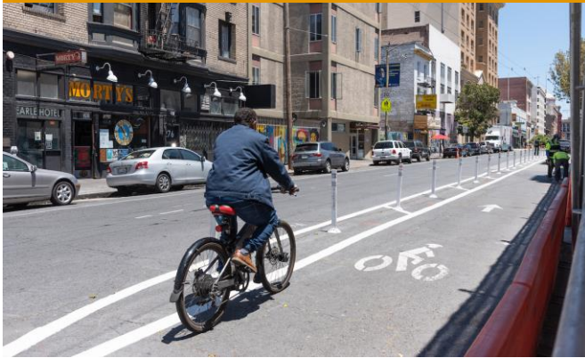
Paint, signs, and delineators
