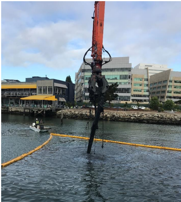
Figure 8: Krypto Klaw removing full steel pile July 17, 2020
