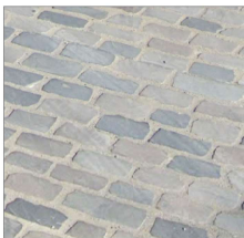
3 cobble w/ compliant walking surface
