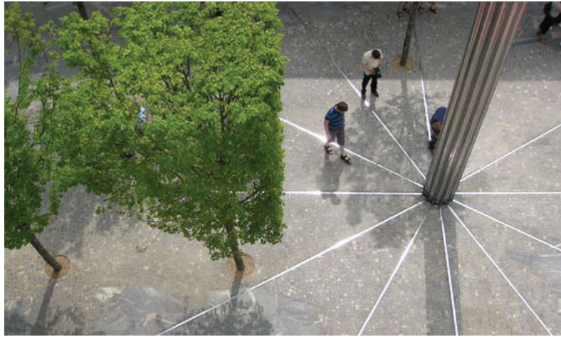
RADIATING METAL INSET PAVING DETAIL
