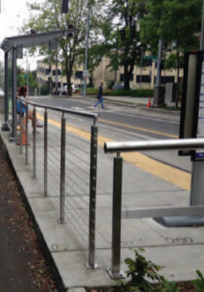
UPGRADED BOARDING PLATFORM
