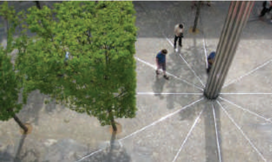
RADIATING METAL INSET PAVING DETAIL
