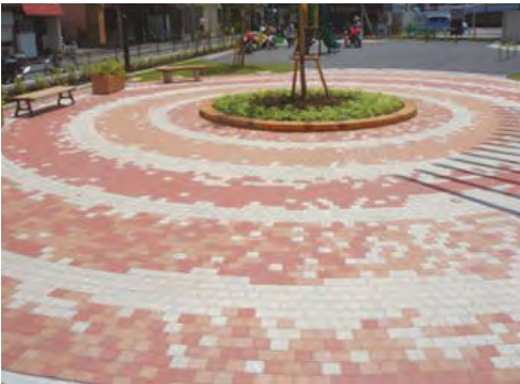
SPECIAL PAVERS IN CIRCULAR BANDS
