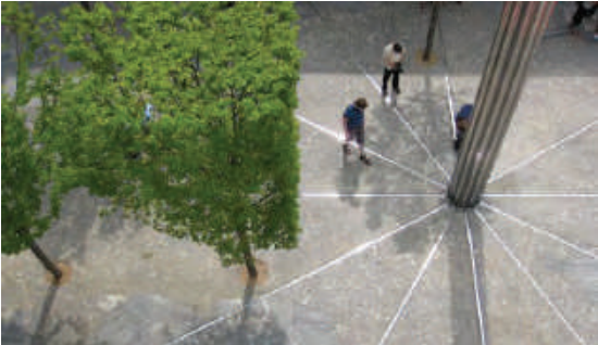
RADIATING METAL INSET PAVING DETAIL
