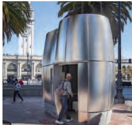
UPGRADED PUBLIC TOILET
