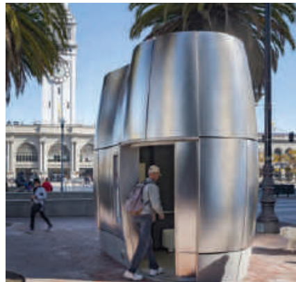
UPGRADED PUBLIC TOILET
