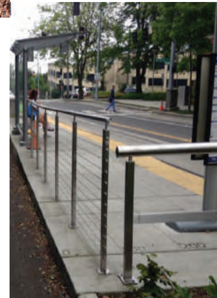
UPGRADED BOARDING PLATFORM
