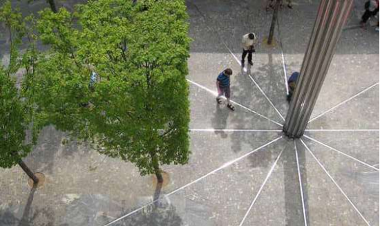
RADIATING METAL INSET PAVING DETAIL
