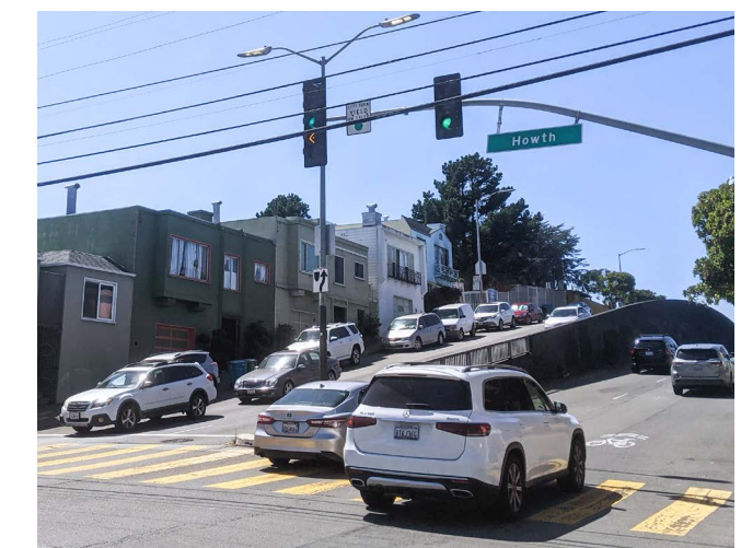
Photo 2: Example of signals on a mast-arm pole aligned to the vehicle lane. (Source: Parisi, 2022)
