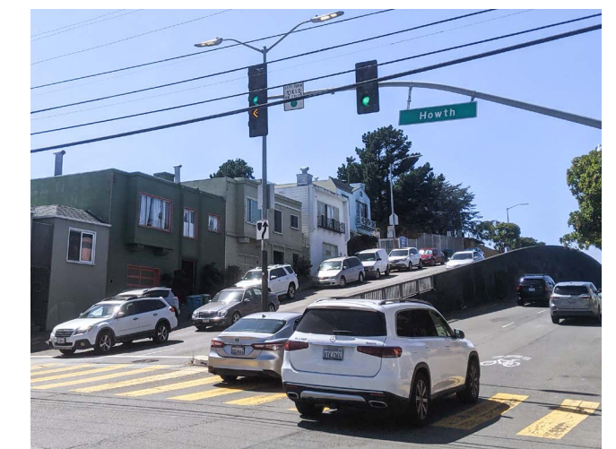
Photo 2: Example of signals on a mast-arm pole aligned to the vehicle lane. (Source: Parisi, 2022)
