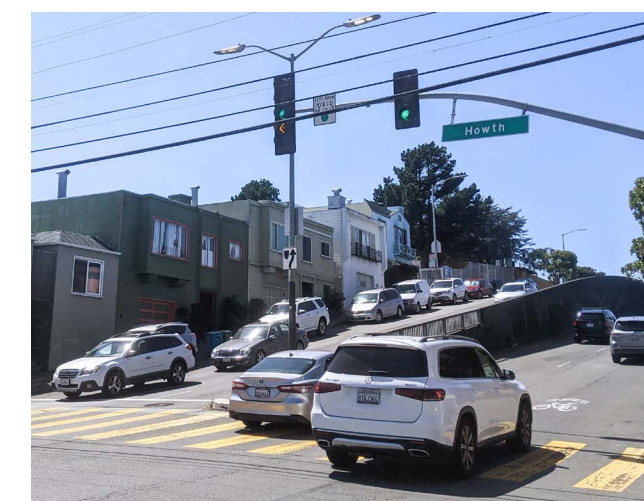
Photo 2: Example of signals on a mast-arm pole aligned to the vehicle lane. (Source: Parisi, 2022)
