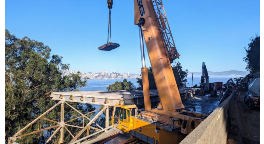
YBI West Side Bridges Project
