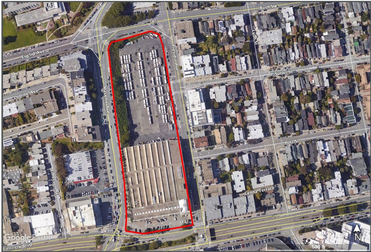
Figure 4-15. Presidio Yard - Existing Conditions (Aerial)
