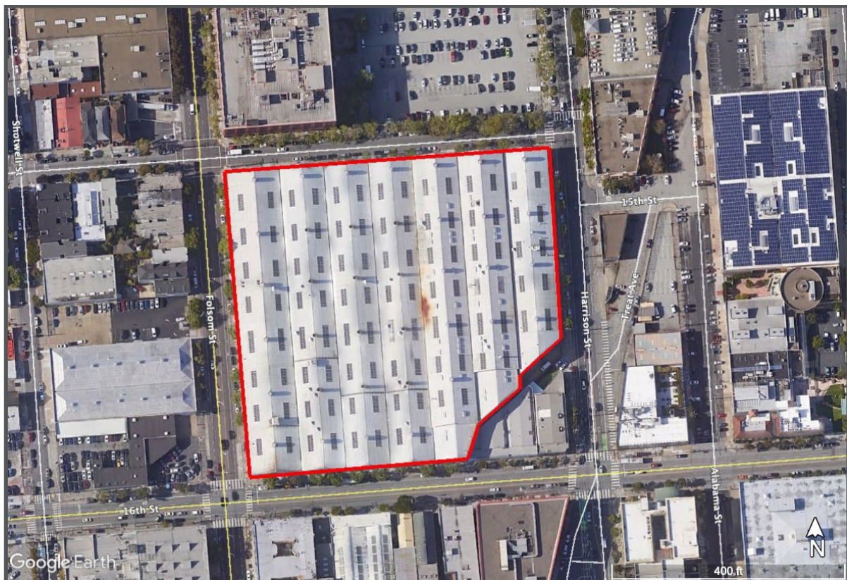
Figure 4-5. Flynn Yard - Existing Conditions (Aerial)
