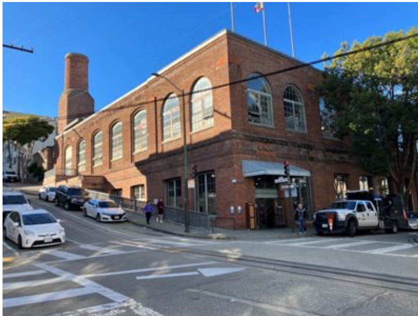
Cable Car Barn & Museum | Exterior View SFMTA Photograph, November 2022
