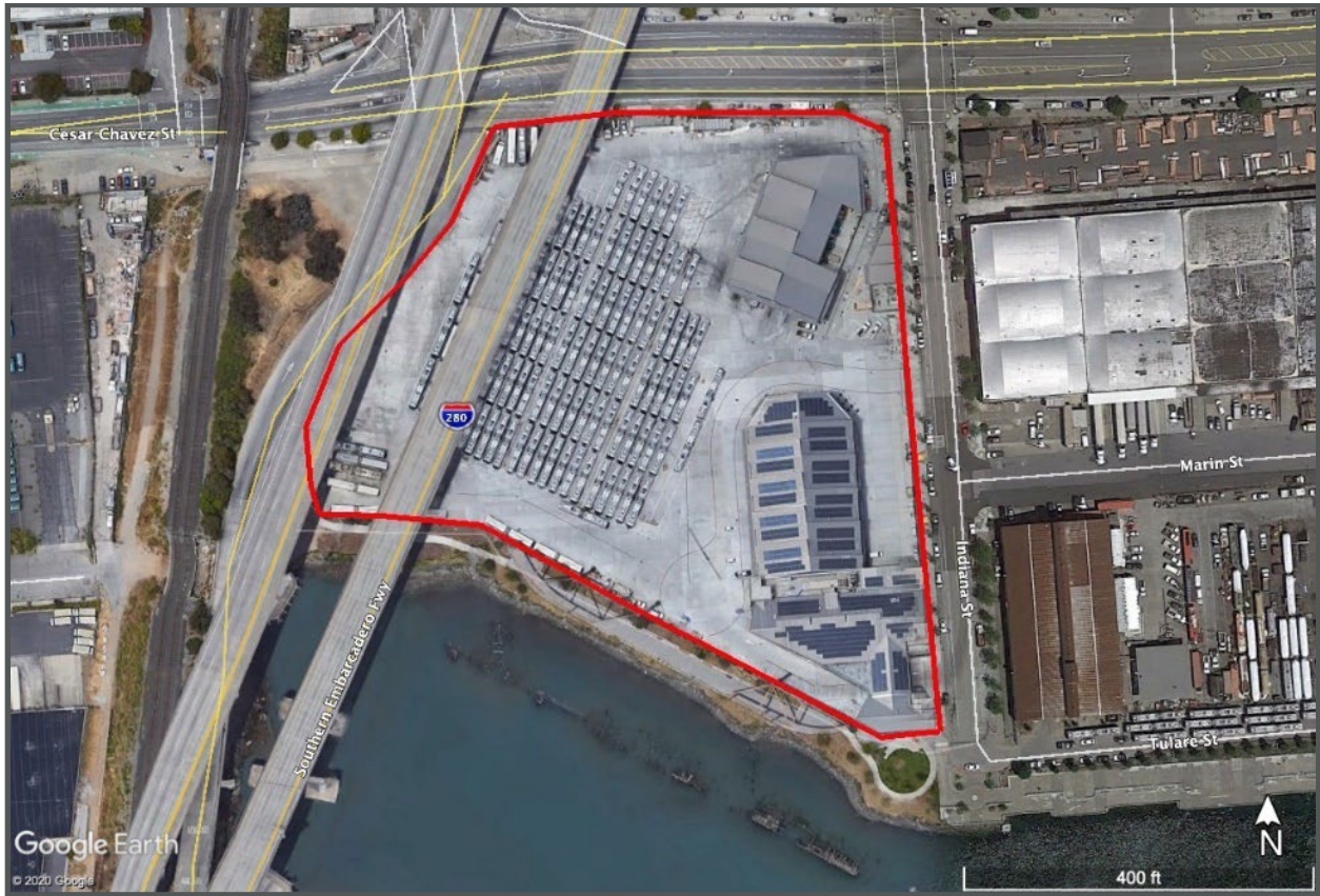
Figure 4-8. Islais Creek Yard - Existing Conditions (Aerial)
