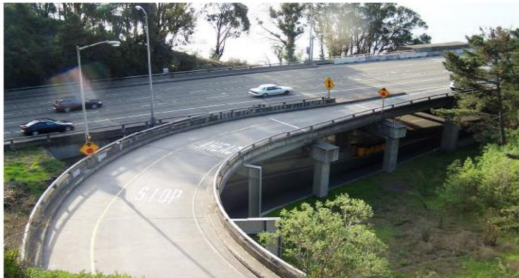
Photo 1: General view of deck.
