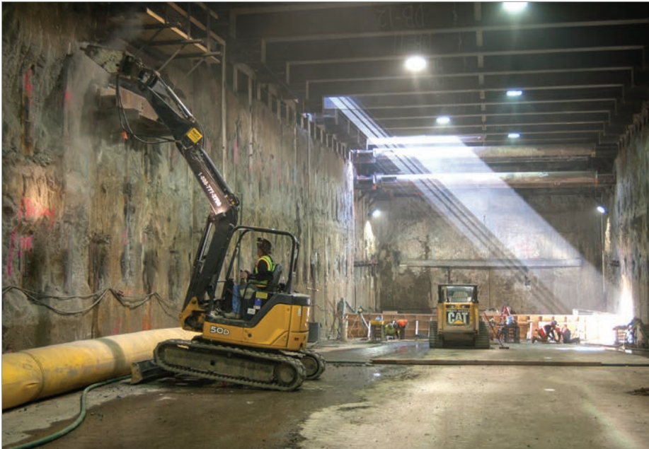
State STIP funds are part of a complex funding plan for the SFMTA’s $1.58 billion Central Subway project. Shown above: constructing the 4th Street launch box for the tunnel boring machines.
