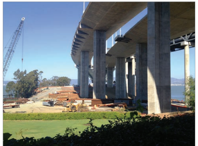
New westbound on and off ramps (on the east side of Yerba Buena Island) will improve access to and from the new Eastern Span of the Bay Bridge.
