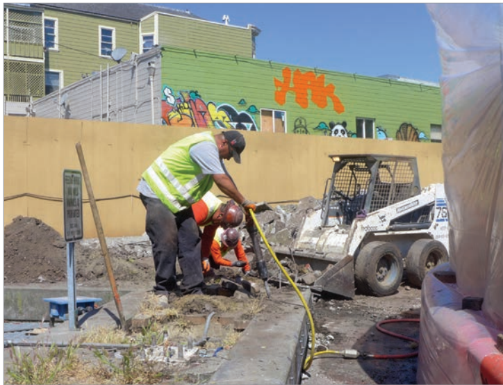
Renovation of the 24th Street Mission BART Station plaza was one of the first projects funded by Prop AA.
