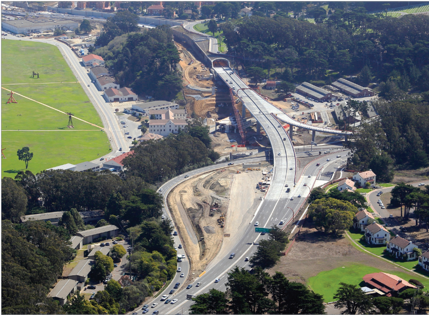
Construction of the Southbound Battery Tunnel and Presidio Viaduct were completed as part of Presidio Parkway Phase I.
