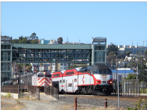
(Top) Moving forward with Positive Train Control: Installation of the Communications Based Overlay Signal System wayside components started in September 2013. (Bottom) The current diesel trains will be replaced by electric multiple units (EMUs).
