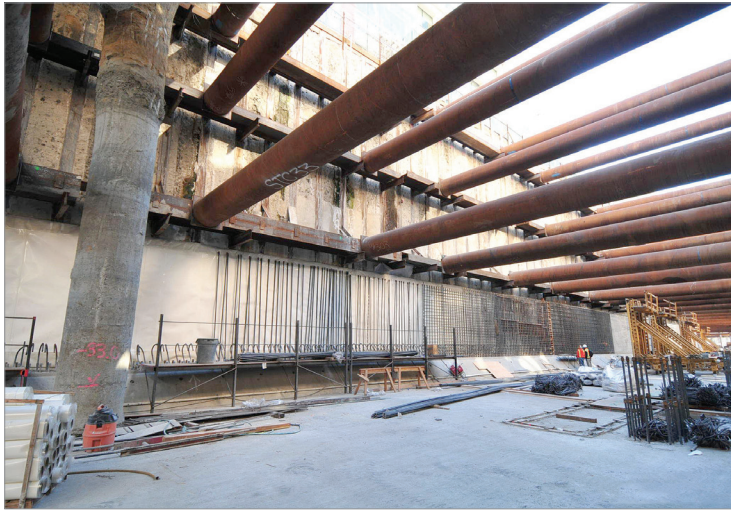
Excavation of the four-block Transbay Transit Center site will be completed in early 2014.
