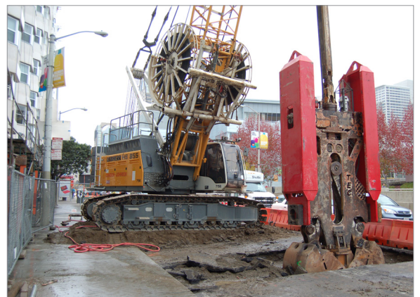
(Top) The cutterhead for "Mom Chung," the first of two tunnel boring machines, being lowered into the 4th Street launch box for assembly. (Bottom) Excavation for the headwalls of the Yerba Buena/Moscone station.
