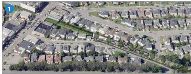
Portal in Lakeside private right-of-way, just south of St. Francis Circle.
