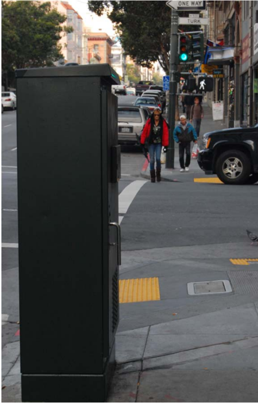
Traffic Controller and new curb ramps
