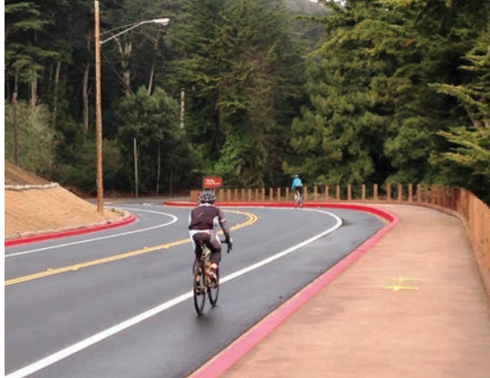
Prop AA funds smaller, high-impact projects throughout the city. The Presidio Trust’s Arguello Gap Closure project addresses gaps in the pedestrian network with a new path, increasing safety for people walking and on bikes.
