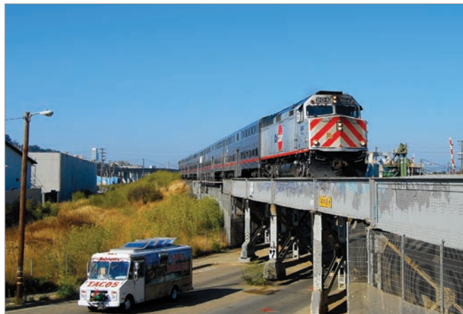
Caltrain will replace this aging bridge over Quint Street. On the adjacent vacant land, the City will construct a new local street connecting north to Jerrold Avenue.
