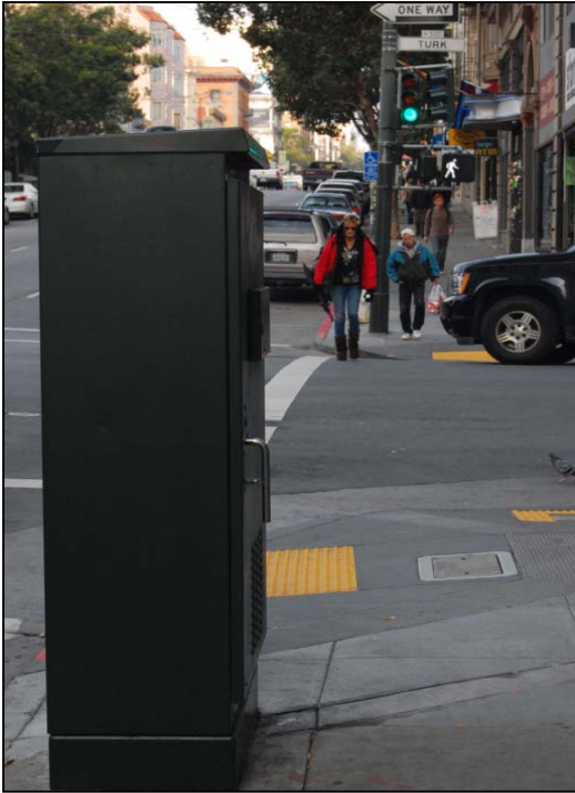
Traffic Controller and new curb ramps
