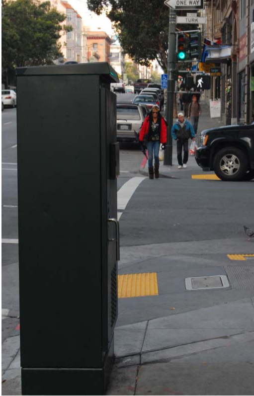
Traffic Controller and new curb ramps
