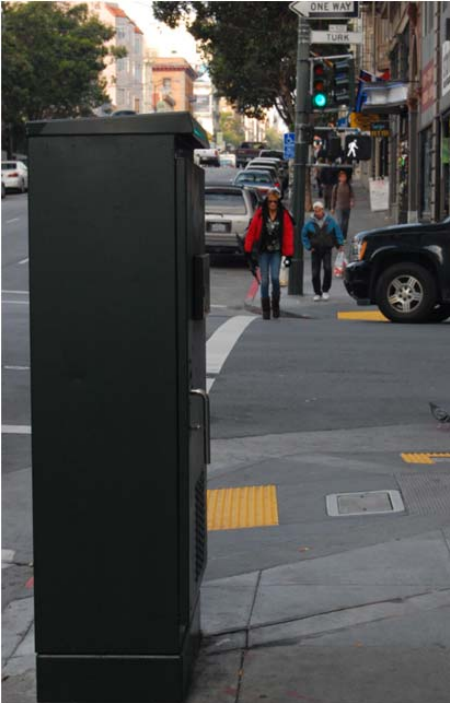
Traffic Controller and new curb ramps
