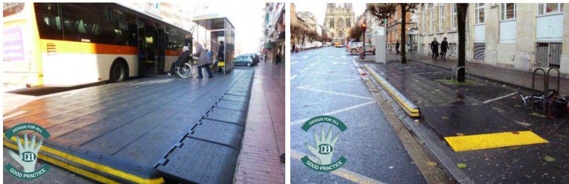
Figure A3-14 Zicla Bus Boarder – Curb Extension
