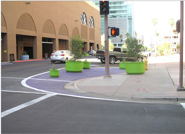
FIGURE 2-4. NON-INFRASTRUCTURE BULB OUTS IN DOWNTOWN PHOENIX
