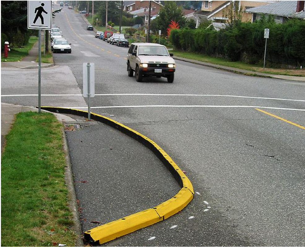
Figure A3-13 Curb Extension using Temporary Materials
