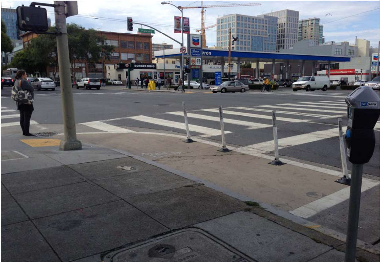
Figure 3. Example of a Painted Safety Zone (PSZ) at Howard Street in San Francisco.
