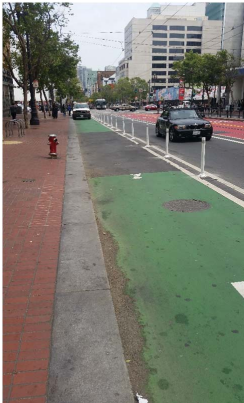
Market Street Bike Lane
