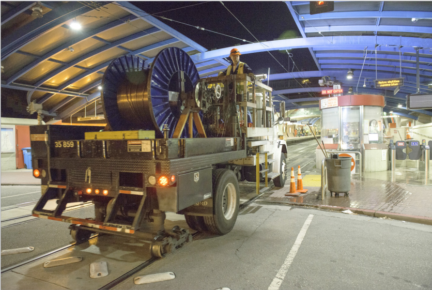
SFMTA radio replacement work is entering the final phases. ▲
