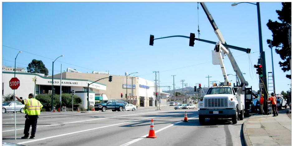
New signal installation is part of the 19th Avenue Combined City Project. ▲
