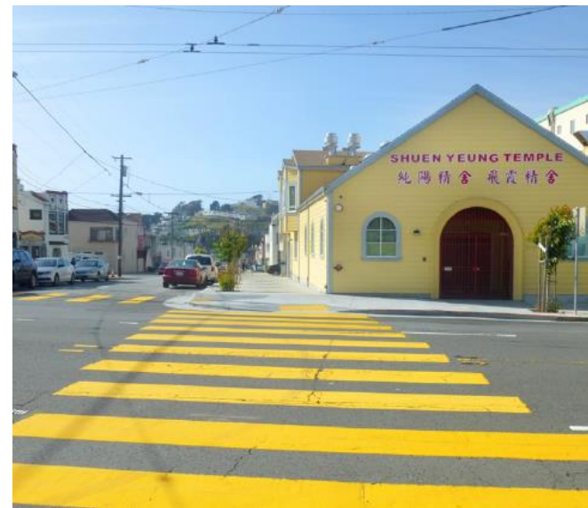
Photo: Pedestrian improvements completed near Longfellow Elementary School
