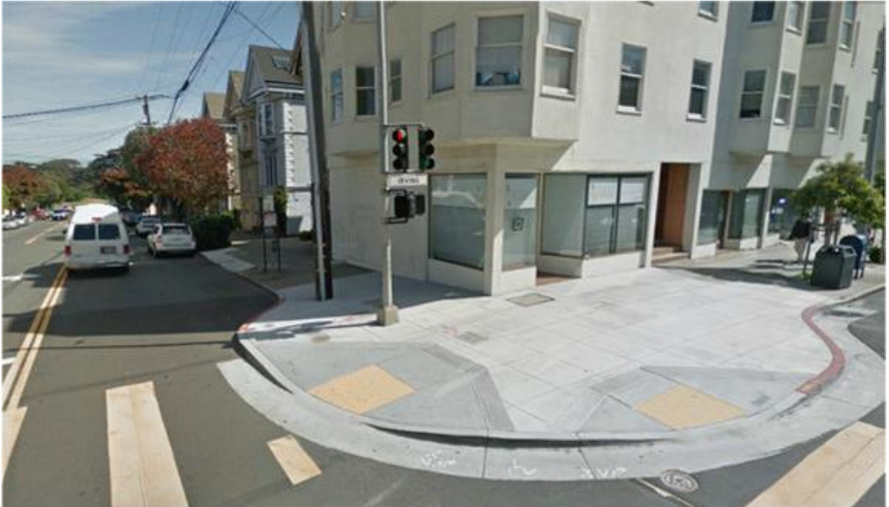
Typical After – Bulb-out
