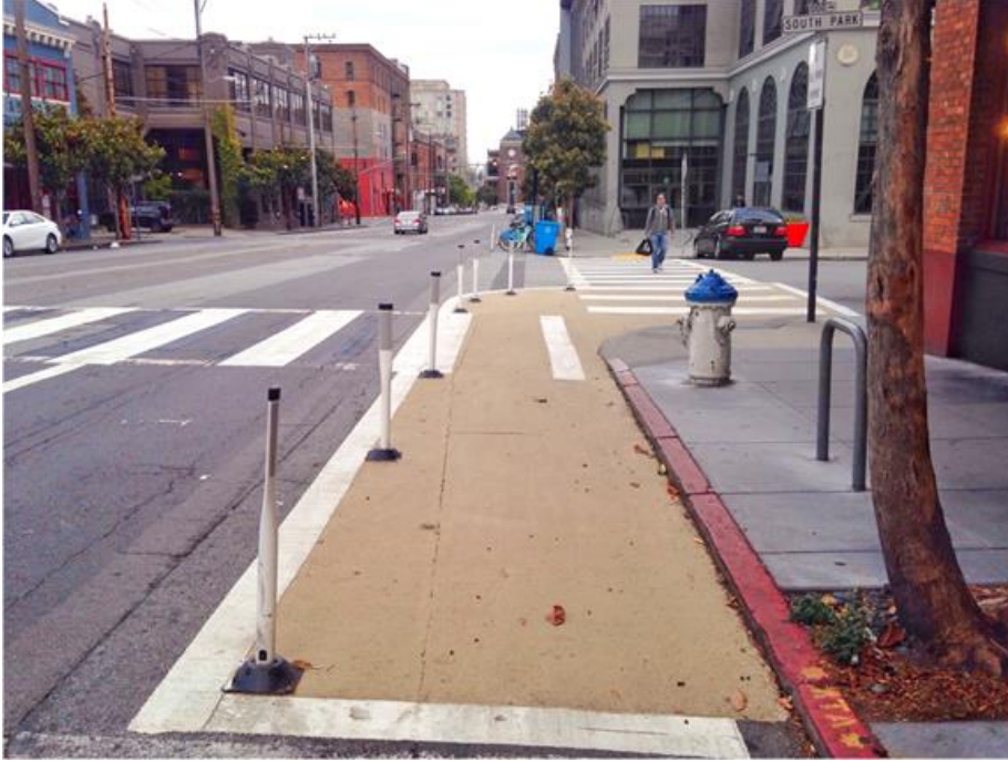
Typical Before – Painted Safety Zone
