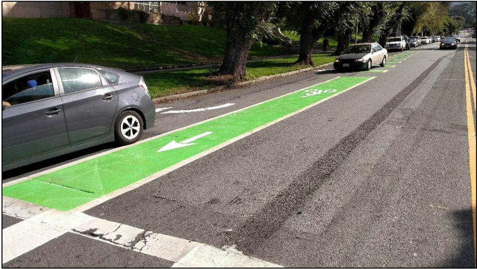
Green bike lane/mixing zone at the intersection of Arguello and Anza
