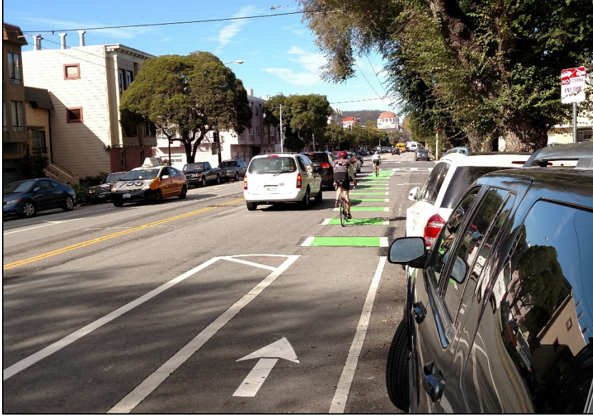
New buffered bike lane and green mixing zone treatment
