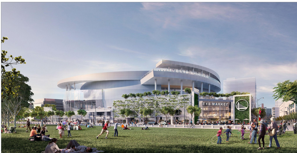
FIGURE 2. The Golden State Warriors arena, now under construction.
