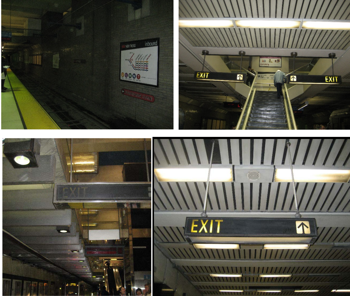
Figure 2: Examples of Lighting Levels and Existing Fixtures
