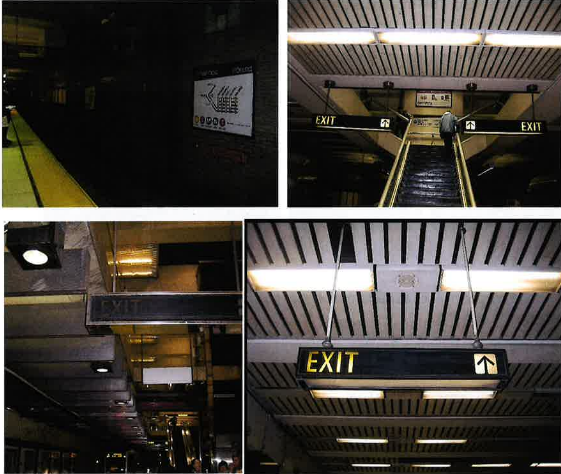
Figure 2: Examples of Lighting Levels and Existing Fixtures
