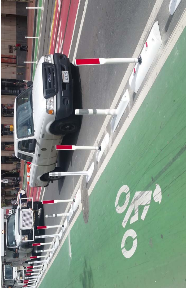
Market Street Delineator w/Curb Pilot Test
